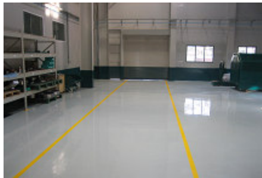
Fig4. Epoxy flooring done by the CONCEPT group.
