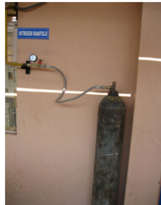
Fig9.; Nitrogen Mnifold.
