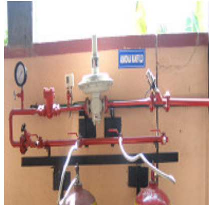
Fig8. Ammonia Manifold.
